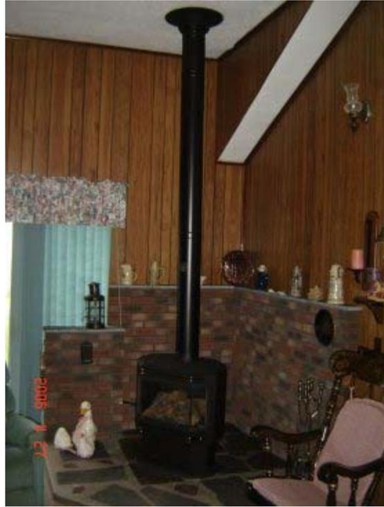
**Above:** After picture of gas stove with vertical vent connecting to the pre-existing Class A chimney that was installed for the wood stove.
