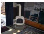
**Above:** In corner with matching Ivory vent pipe paint. Horizontally vented through sidewall. Standard cap on outside.
